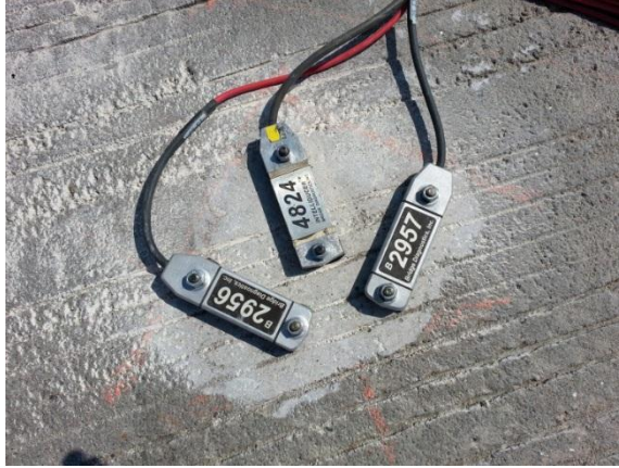
Figure 5. Rosette near b2 reinforcement
